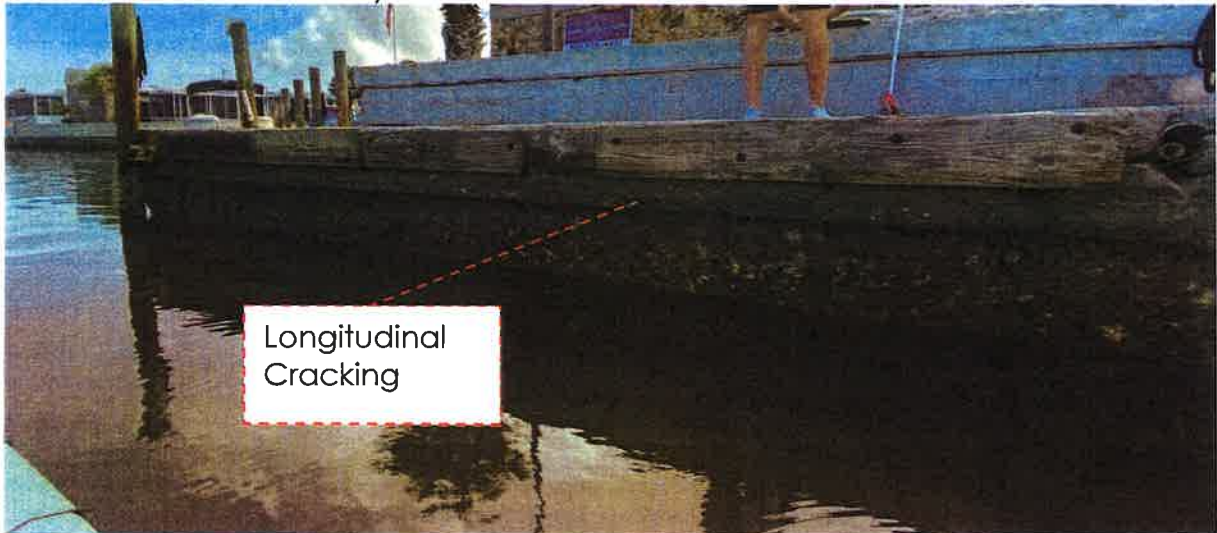
Photo #1- View of Wall by Marina.
